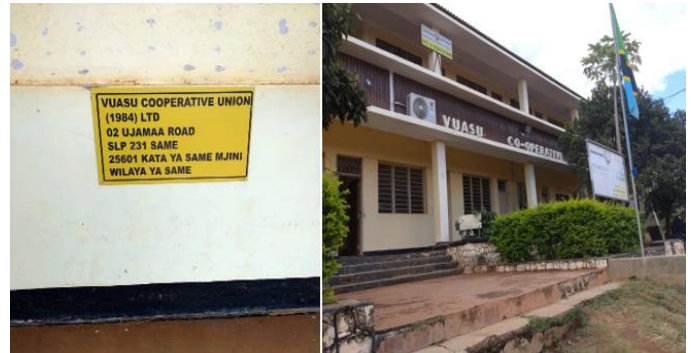
Figure 2. VUASU Co-operative Union (VCU) headquarters in Same District, Kilimanjaro Region. The administrative building and signage are interpreted as reflecting its historical role in supporting cooperative agricultural systems. Photo by author.
